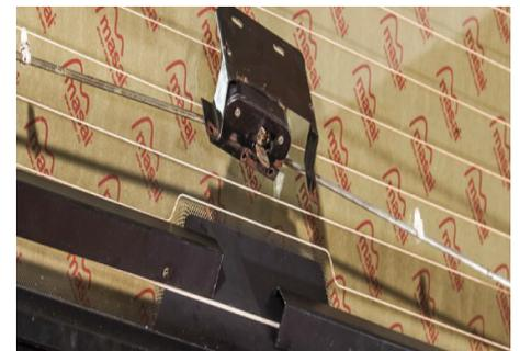
19. Next, connect the catch actuator rods, and drill the covers. Leave the covers off, as you will need to access the rod locknuts later.
