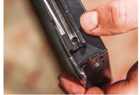
14. On the lower edge, fit the rubber seal retainer with screws or rivets. The deeper return (indicated with screwdriver) should face the outside edge.
