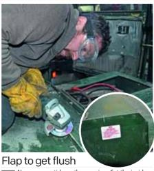
Now you can tidy up the opening. Cut the inside top corners off to match the shape of the riveted ridge. Trim the lower edge 2mm to 3mm above the floorpan. To get this completely flush, and to de-burr all the edges, use a flap disc.
